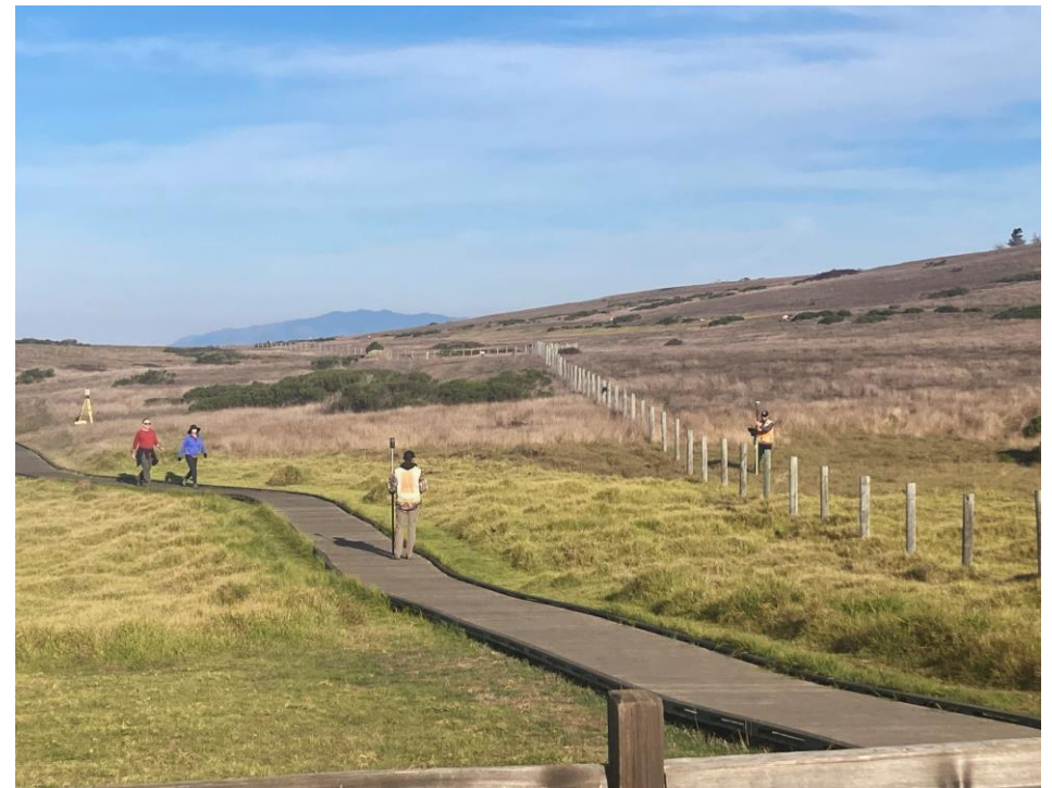
Engineers surveying the new boardwalk alignment.
